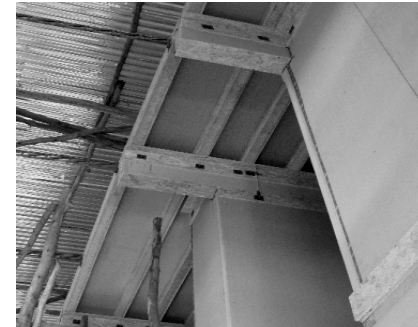
SECU – first floor with cantilevered roof (three days)
