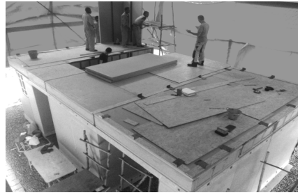
SECU – placing of hollow core slabs (two days)
