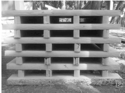
SECU - Prefabricated roof elements made of two layers of straw boards
