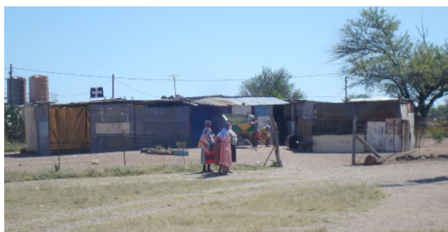
Fig. 9. Shelter in cut metal sheets. There is water and electricity. Source: Author's Photo
